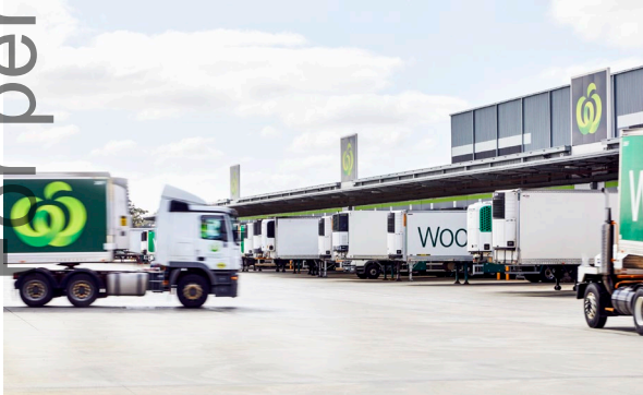
Woolworths Distribution Centre, Melbourne
