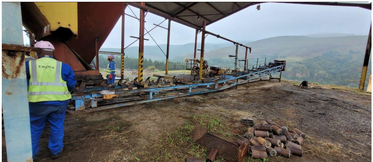
Figure 11: Removal of old conveyor belt structure
