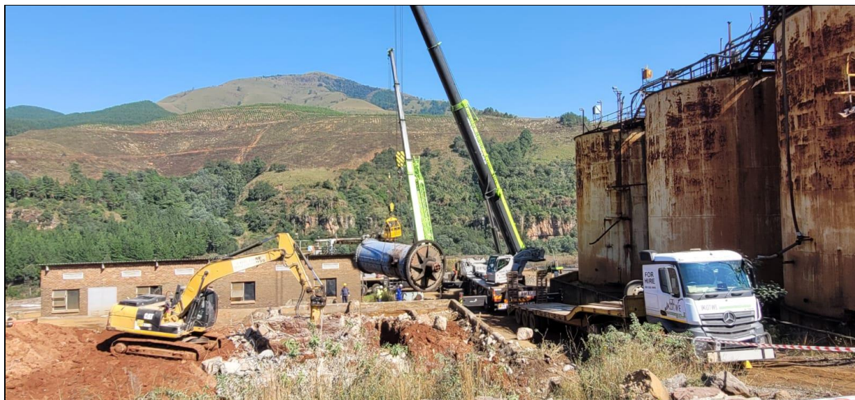
Figure 5: Breaking of old mill civils and loading of ball mill
