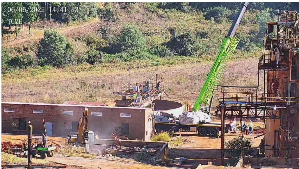
Figure 1: Demolishing and removal of old equipment
