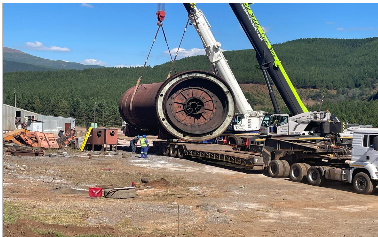
Figure 6: Lifting and loading of the big ball mill for transport to the laydown area
