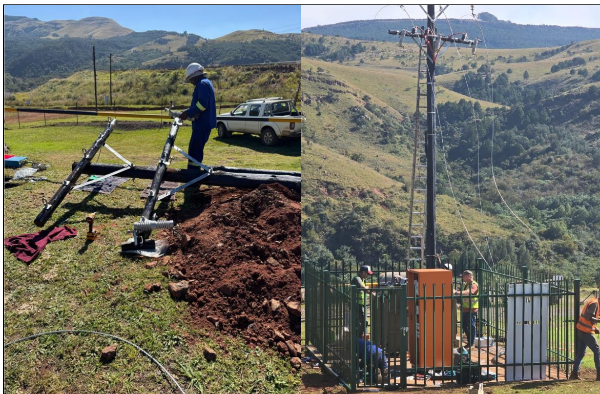
Figure 4: Installation of temporary electrical plant supply
