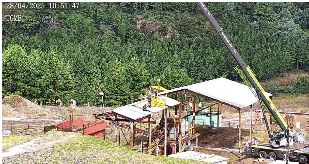
Figure 9: Removal of old mill sections
