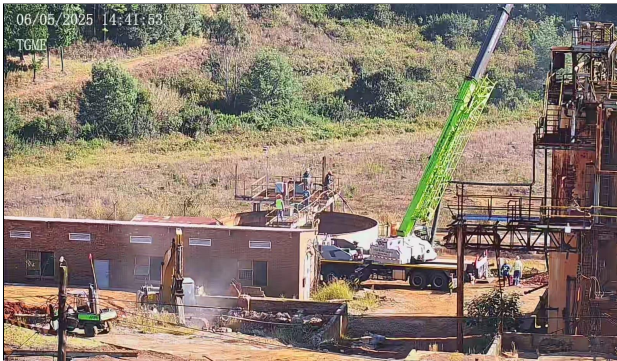
Figure 3: Removal of old mill civils and thickeners
