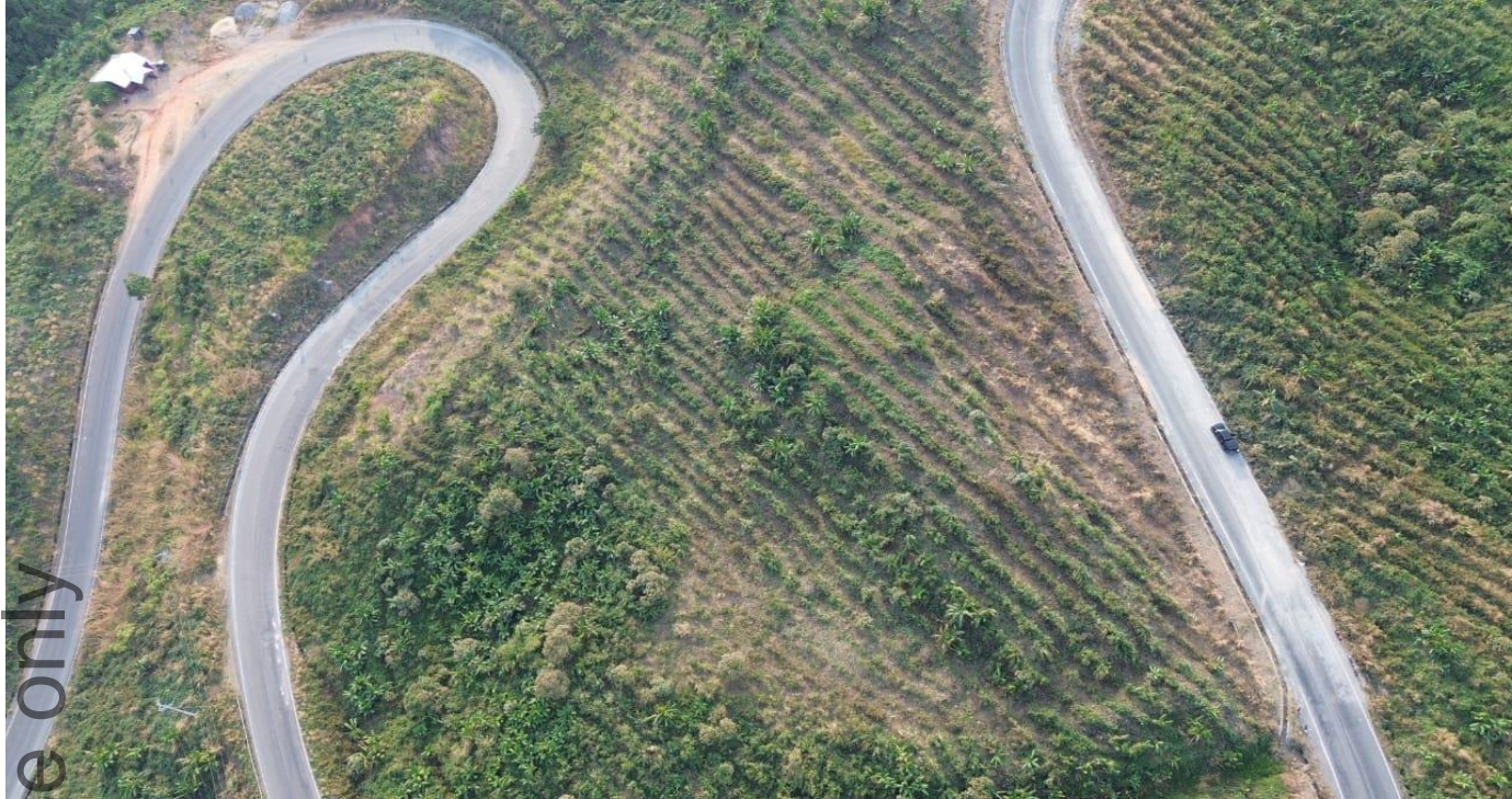
Figure 19 | Regular dry-season maintenance successfully removes overgrowth from trees to promote healthy growth at Phnom 1500
