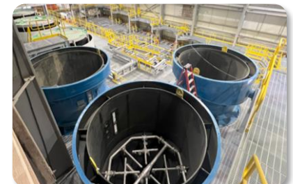
Interior work - South
