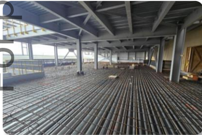
Interior structural work
