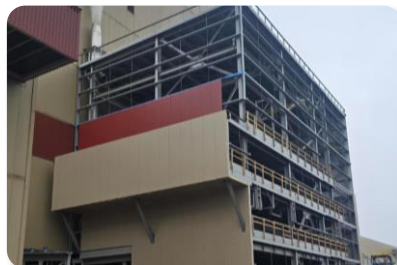
Structural work - North
