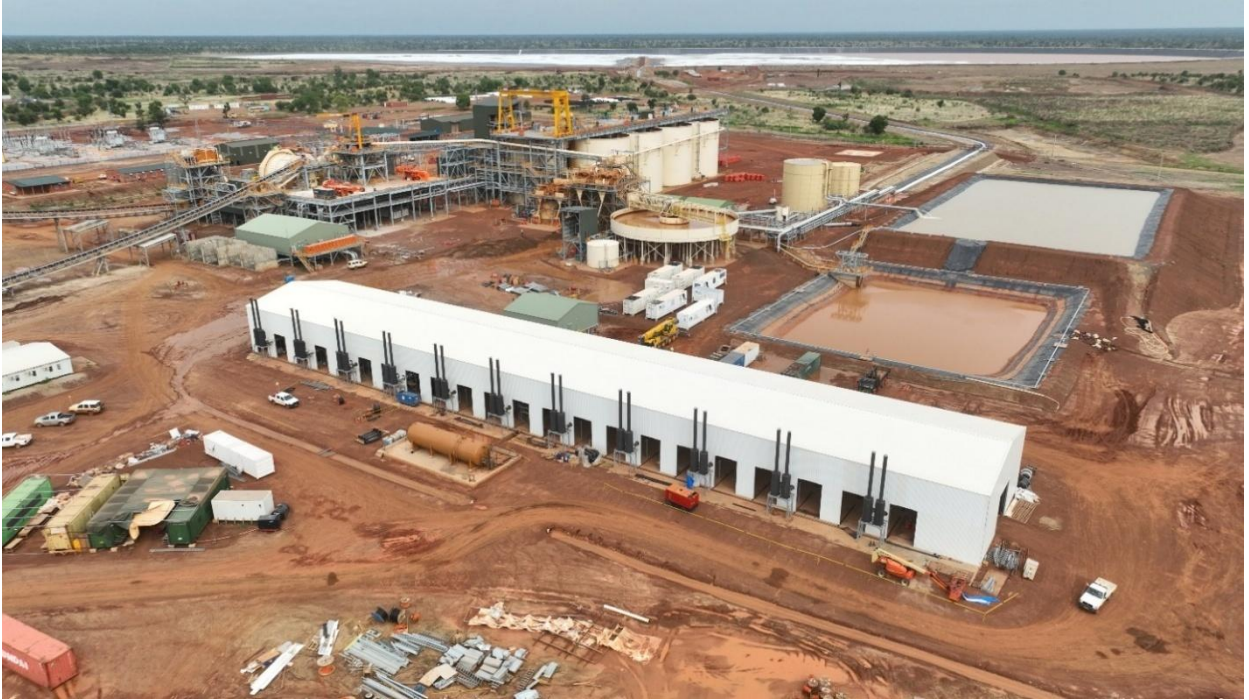
Kiaka Plant with Generator Shed in Foreground
