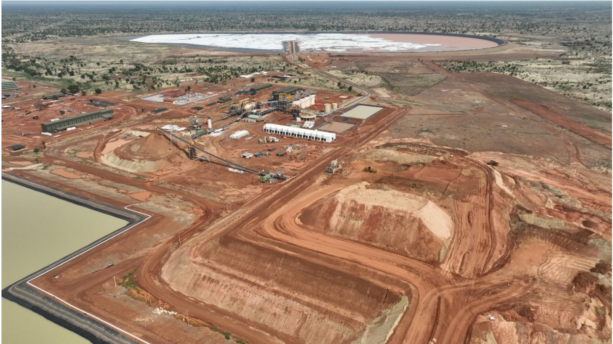
Kiaka Plant Overview with ROM Pad in Foreground and TSF in Background
