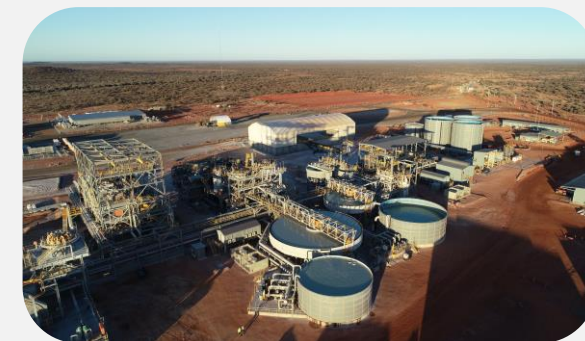
Aerial view of plant
