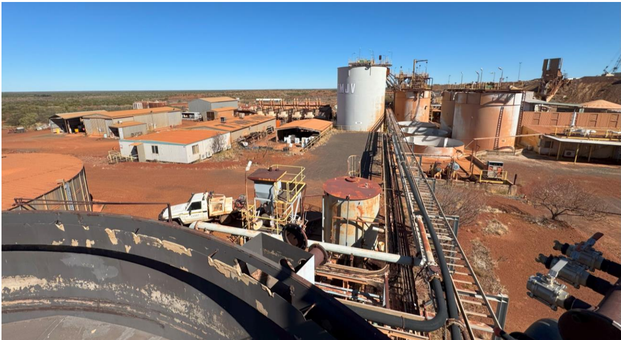
Figure 2 CTPJV 1.2 Mtpa Processing Plant (idle since 2005, requires refurbishment)
