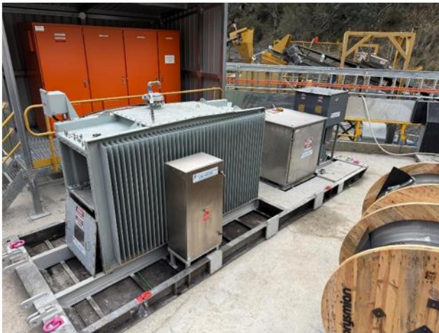
Figure 1 – High voltage (415V to 11kV) transformer installed next to power station at the Reward Gold plant
