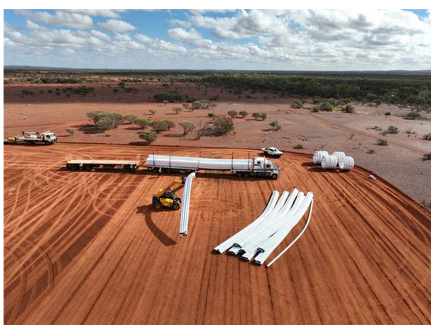
Figure 2 – Water pipeline being unloaded
