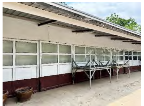
View of the single-storey warehouse 1
