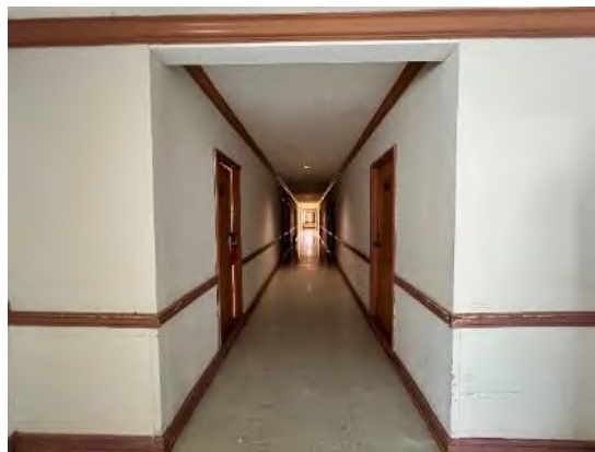
Internal view of the single-storey hotel (Hotel 113)
