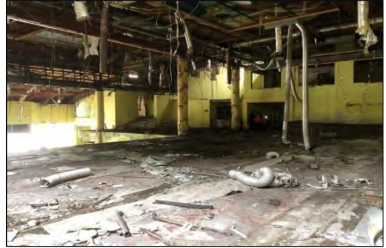
The Property– Internal View
