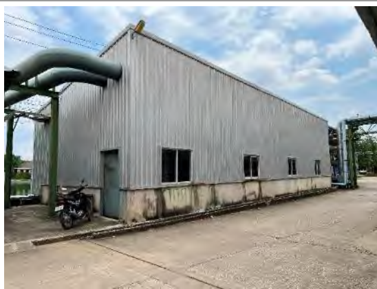
View of the single-storey water chiller building
