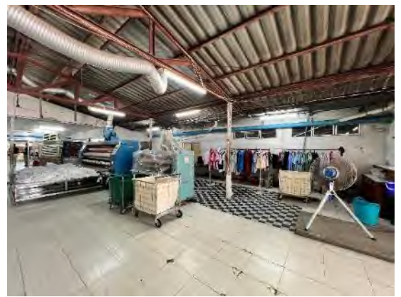
Internal view of the single-storey laundry building
