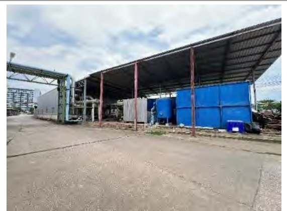
View of the single-storey water chiller building
