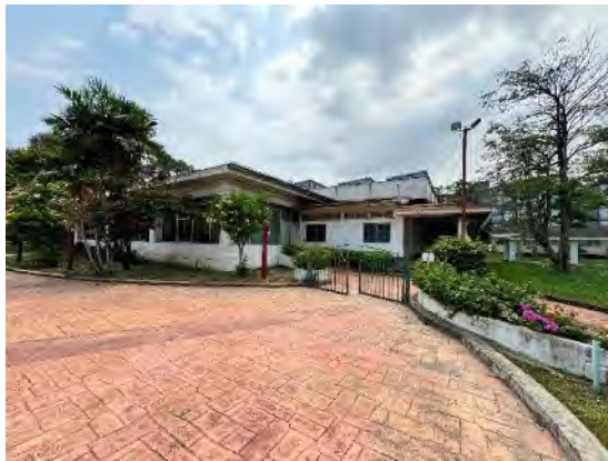
View of the single-storey gymnasium
