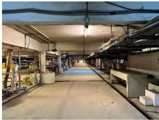
Internal view of the double-storey casino (Basement)
