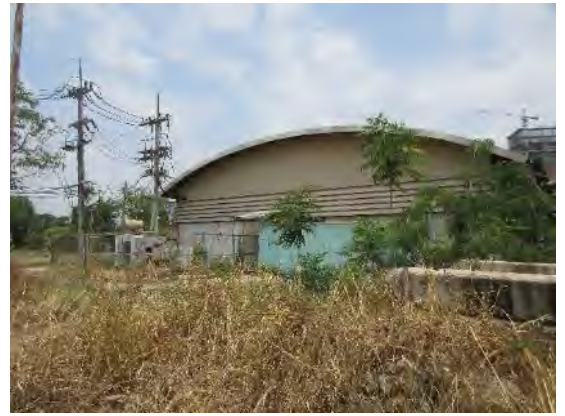
View of the single-storey power plant building
