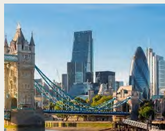
Valuation Leadenhall Building, London
