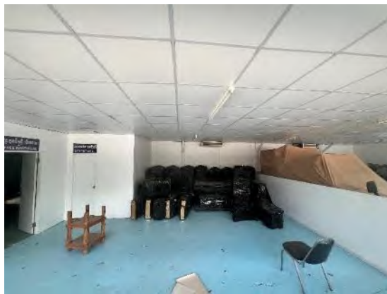
Internal view of the single-storey warehouse 1
