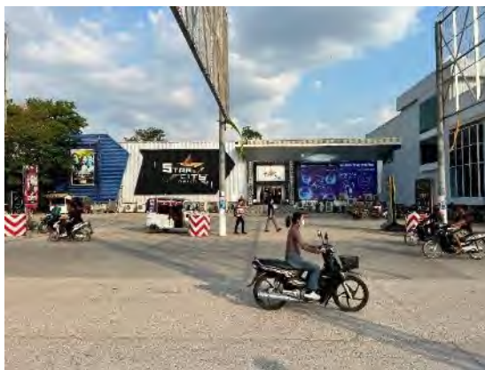
View of the single-storey entertainment building (Star City)
