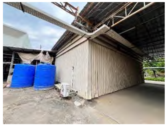
View of the single-storey warehouse 2
