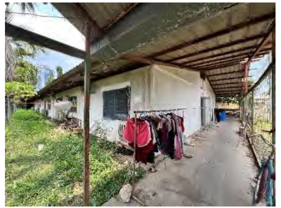
View of the two single-storey residence
