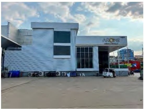
View of the double-storey restaurant
