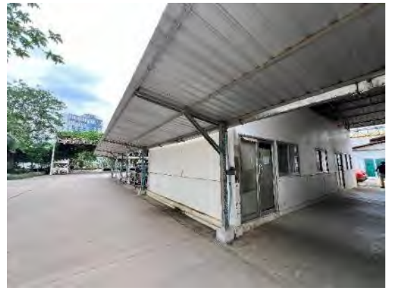
Internal view of the single-storey warehouse 2
