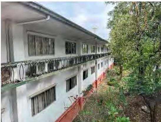
View of the double-storey hotel (Hotel 100)
