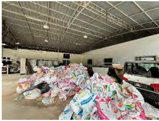
Internal view of the single-storey warehouse 2
