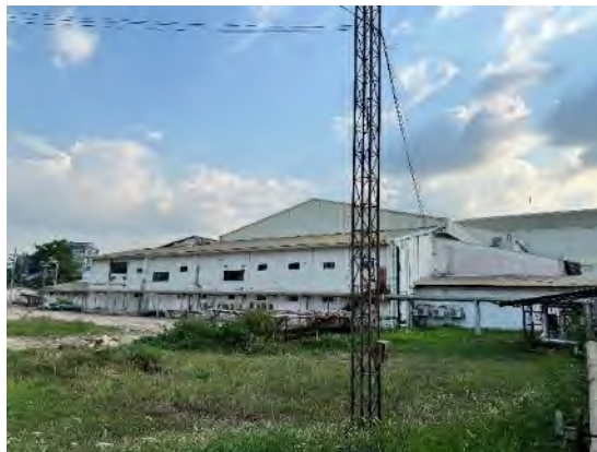
View of the double-storey casino (Casino 2)
