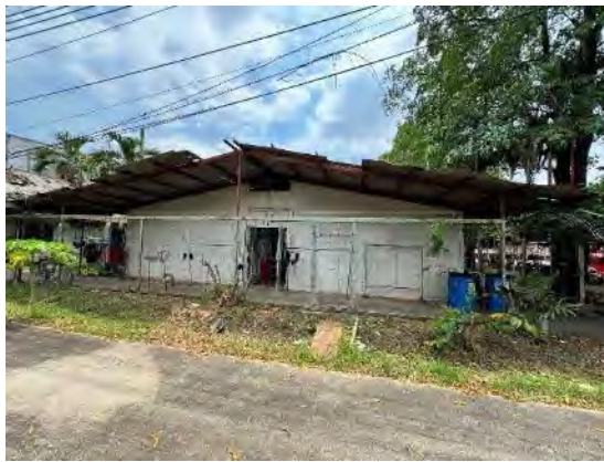
View of the two single-storey residence
