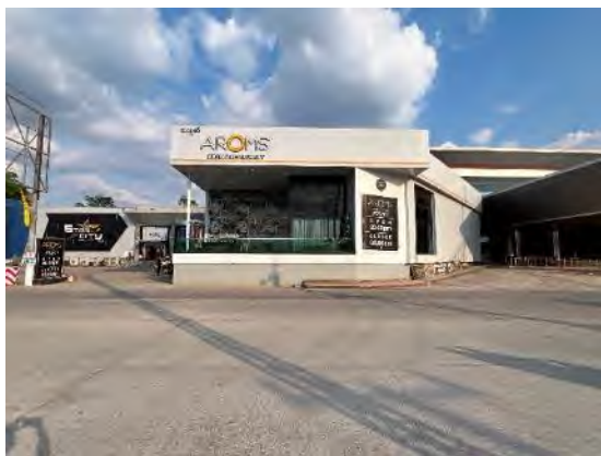
View of the double-storey restaurant
