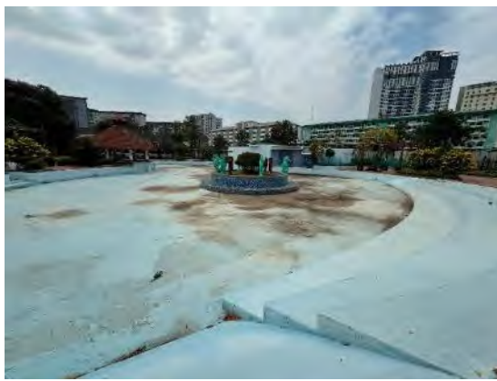
View of the swimming pool
