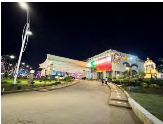
View of the double-storey casino (Casino 1)
