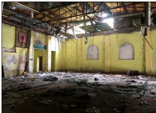
The Property – Internal View
