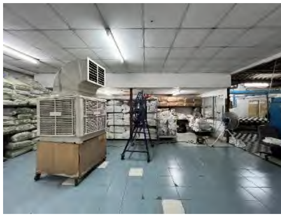
Internal view of the single-storey laundry building
