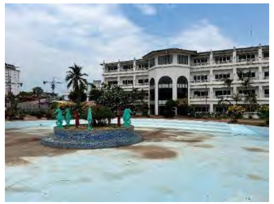
View of the swimming pool
