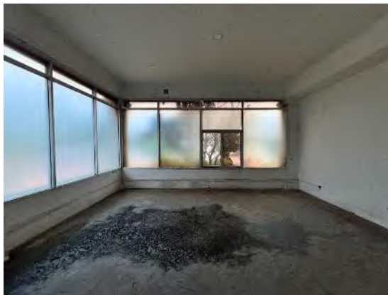
Internal view of the single-storey gymnasium
