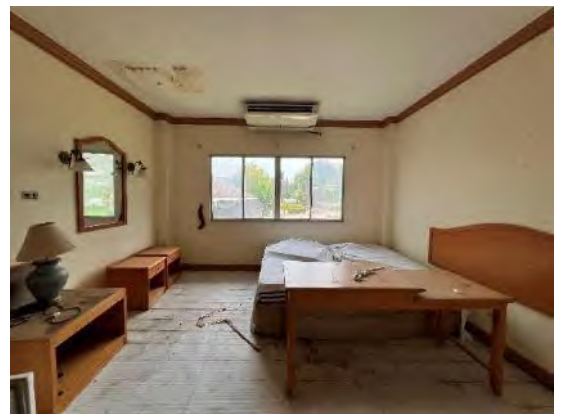
Internal view of the single-storey hotel (Hotel 113)
