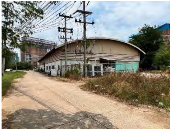
View of the single-storey power plant building
