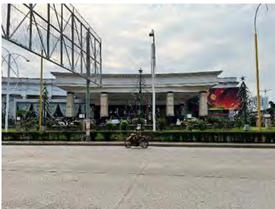
View of the double-storey casino (Casino 1)
