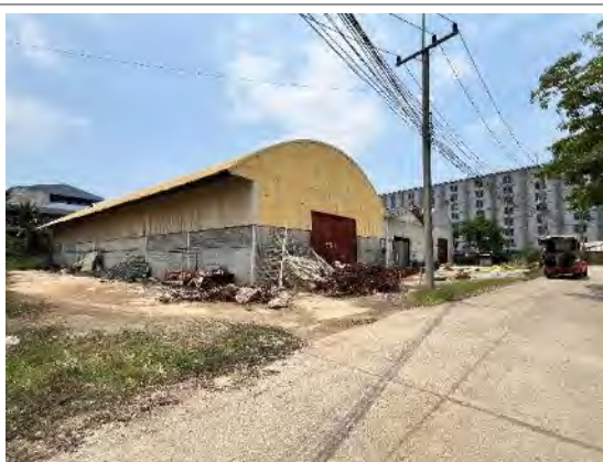
View of the single-storey warehouse 3
