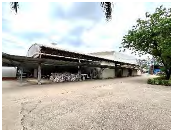
View of the single-storey warehouse 2
