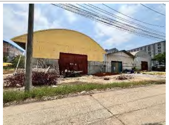
View of the single-storey warehouse 3
