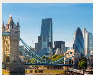
Valuation Leadenhall Building, London
