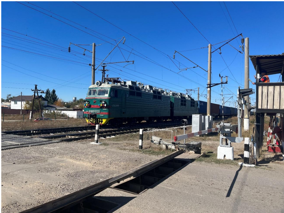
Figure 1 - Electrified heavy haul railway crossing in Agadyr, Kazakhstan
