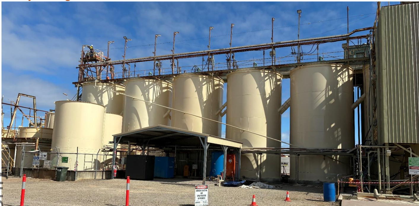
Completed blasting & painting all 6 CIL Tanks
