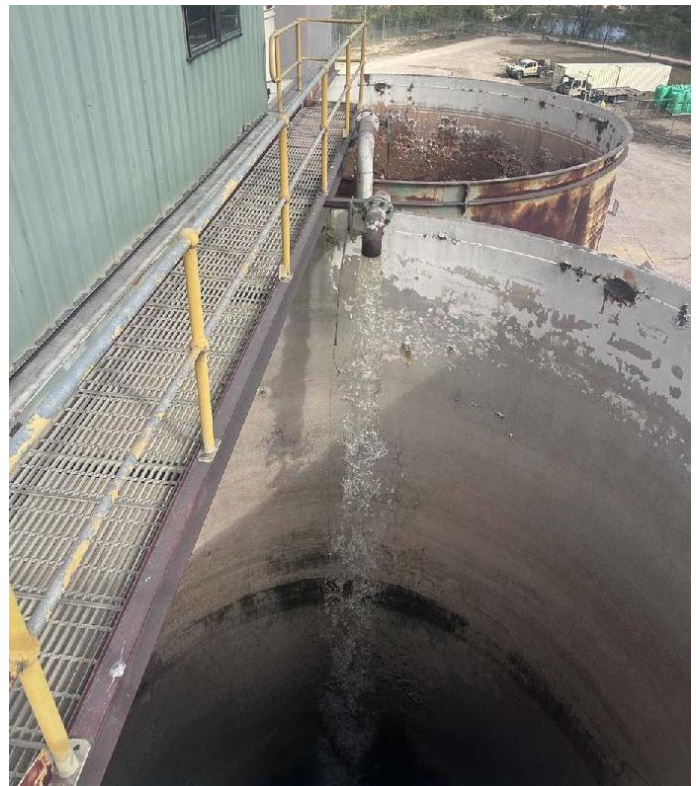
Filling up process water tanks in preparation for plant commissioning
