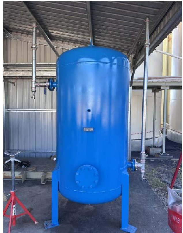
Upgraded and upsized new air receiver
