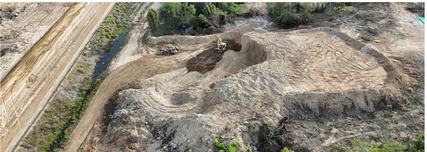
Mixing and blending gravel at Borrowed Area
