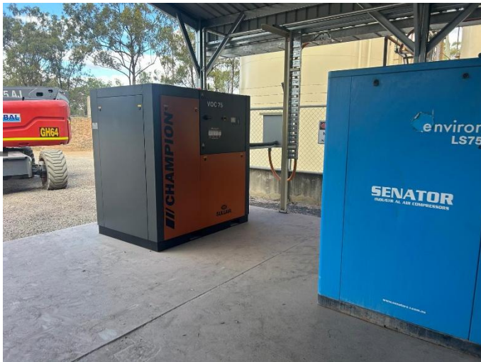
Air compressors installed, ready for Hitachi commissioning
