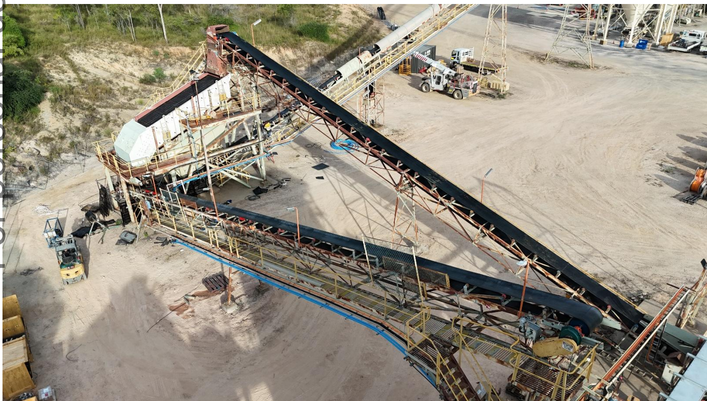
New belts installed for all five conveyors
