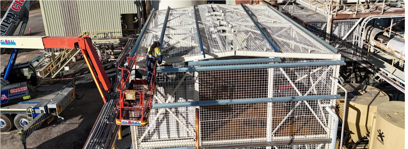
Gold room steel mesh and purlin installation
