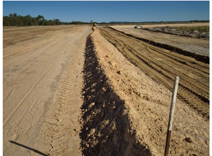
Northeastern wall subgrade finished
