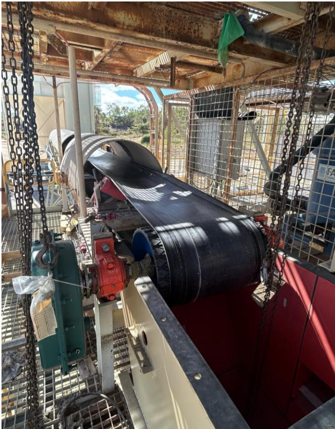
Installation of new belt and internal wear lining completed on the ball mill feed conveyor and feed chute
