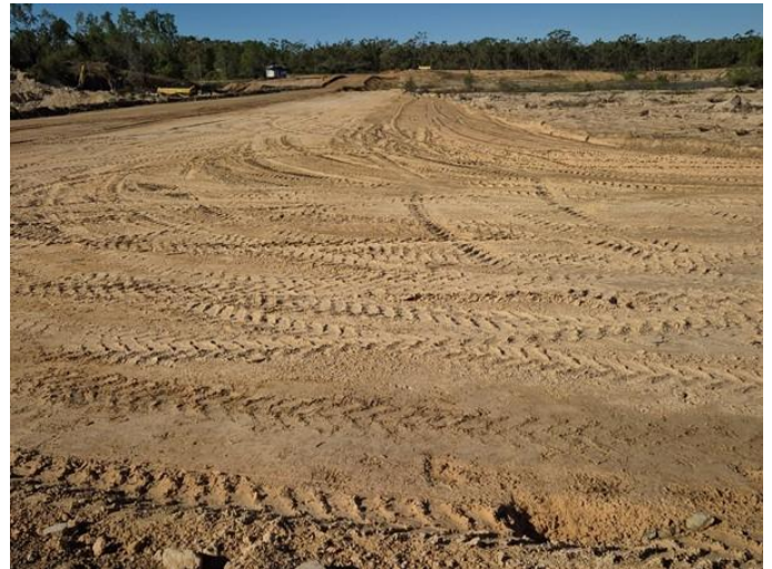
Northwestern wall subgrade finished
