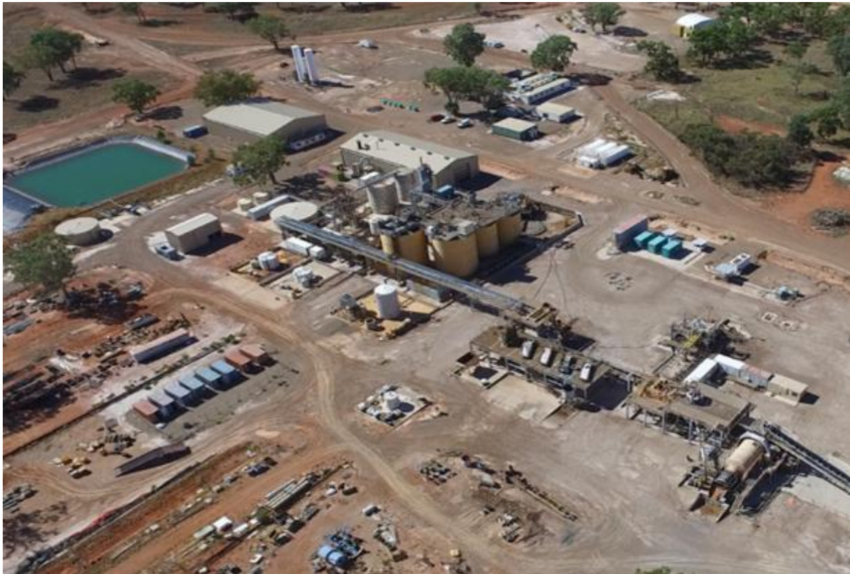
Figure 3: The existing Wonawinta Processing Plant.
