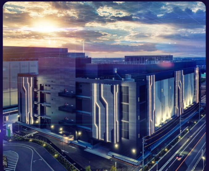
STT Data Centre, Goodman Business Park, Chiba, Japan
