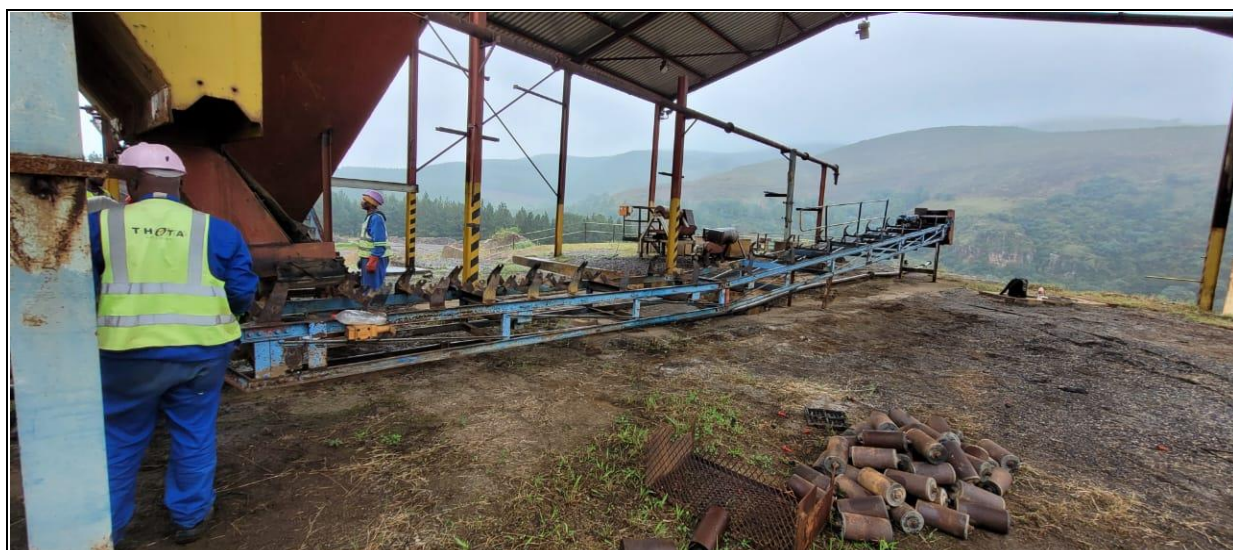
Figure 5: Removal of old conveyor belt structure
