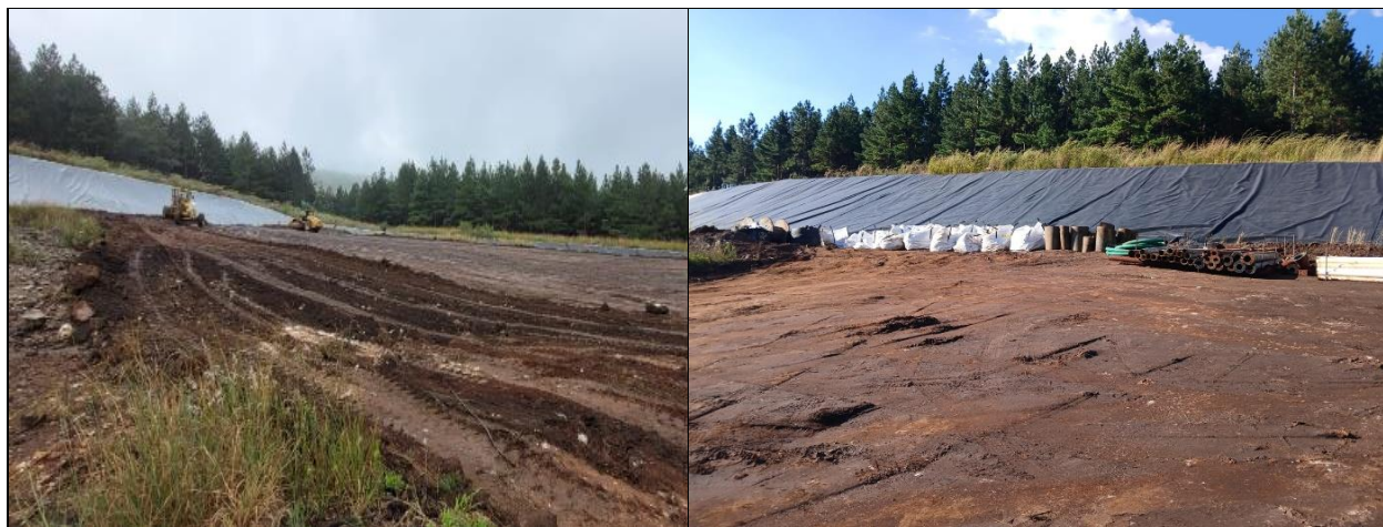
Figure 4: Salvage laydown area
