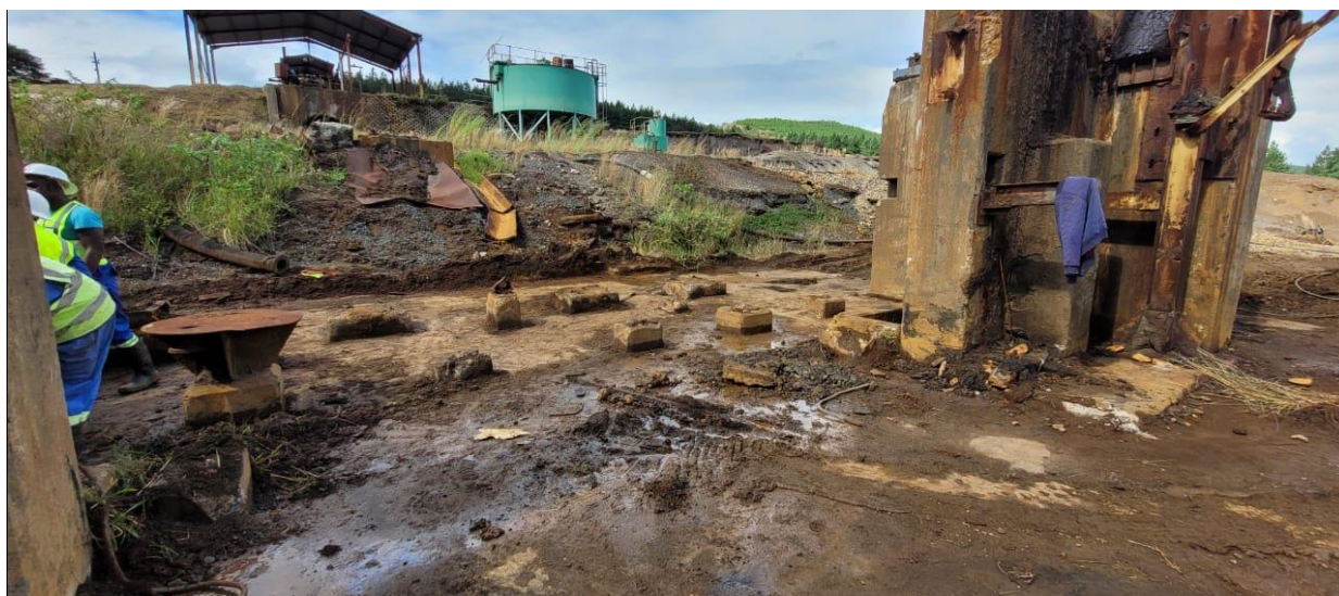
Figure 6: Old mill civils to be removed
