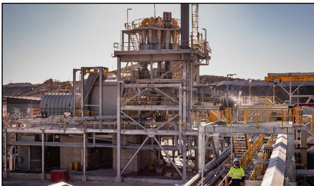
Figure 6: SAG mill in operation
