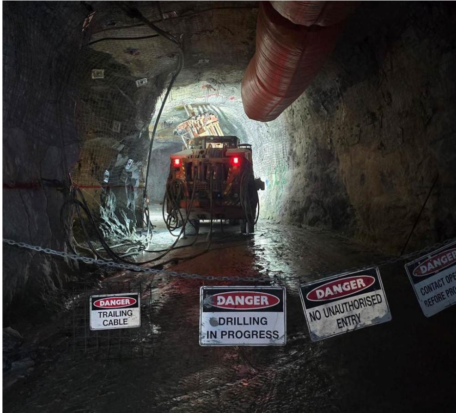
Figure 1: A long-hole drill rig drills upward into the stope's firing zone to prepare for blasting
