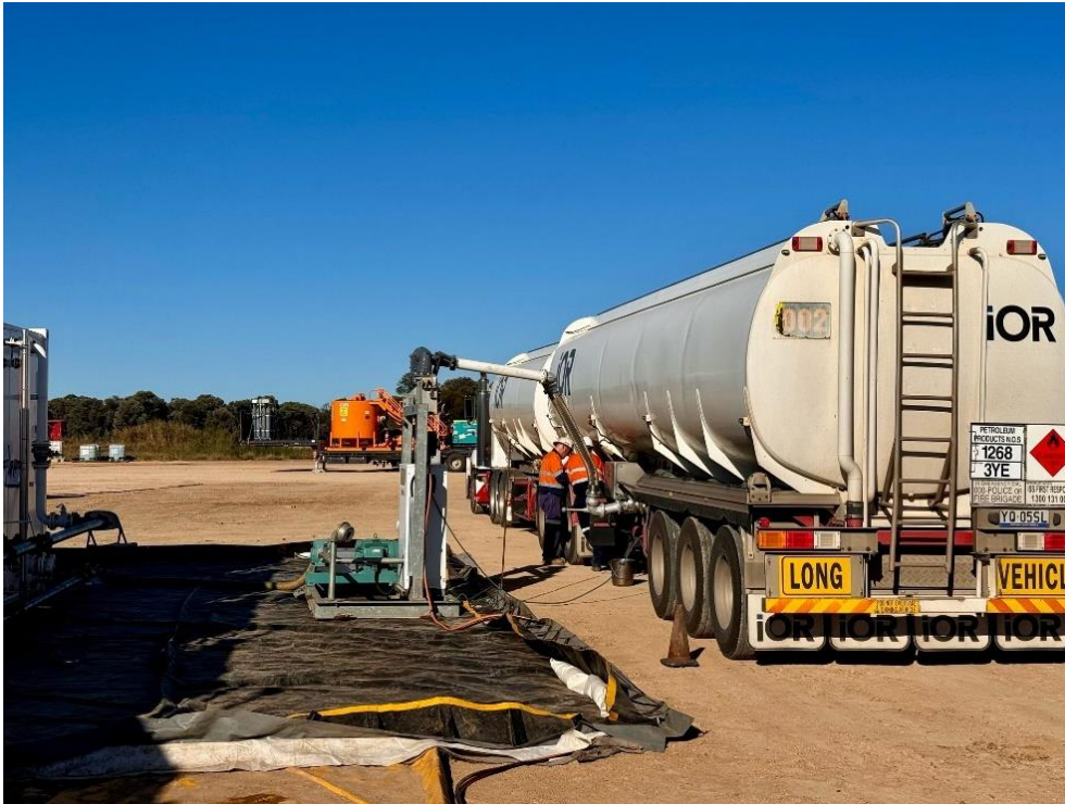
Figure 1: tanker being loaded with oil from the Canyon-1H well for transport to refinery
