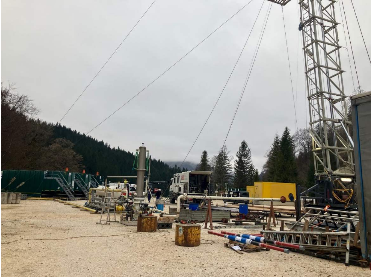
Figure 10: Well completion work and Flow Testing Facilities set up at the Welchau-1 well location
