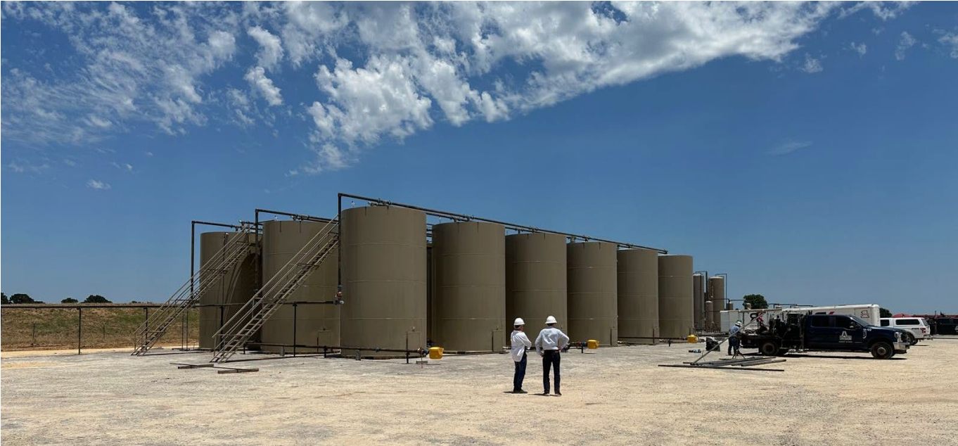
Figure 3: Sanford Pad tank battery at the FMDP project in Carter County, Oklahoma
