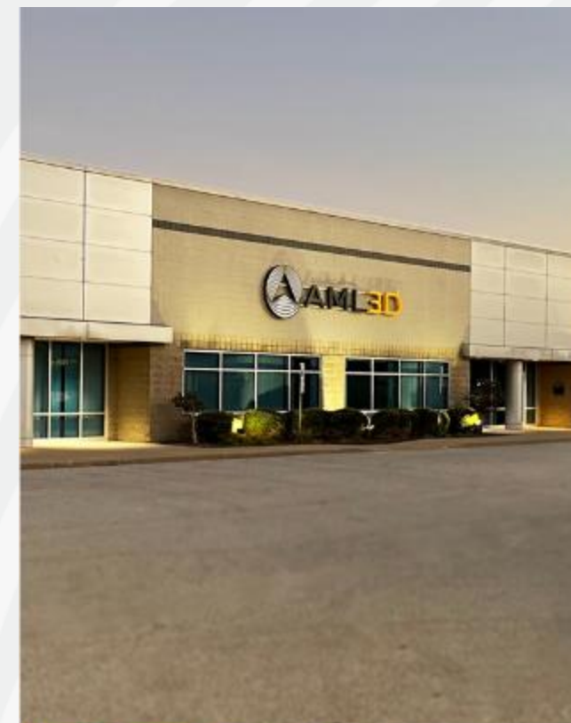
AML3D Stow Technical Facility
