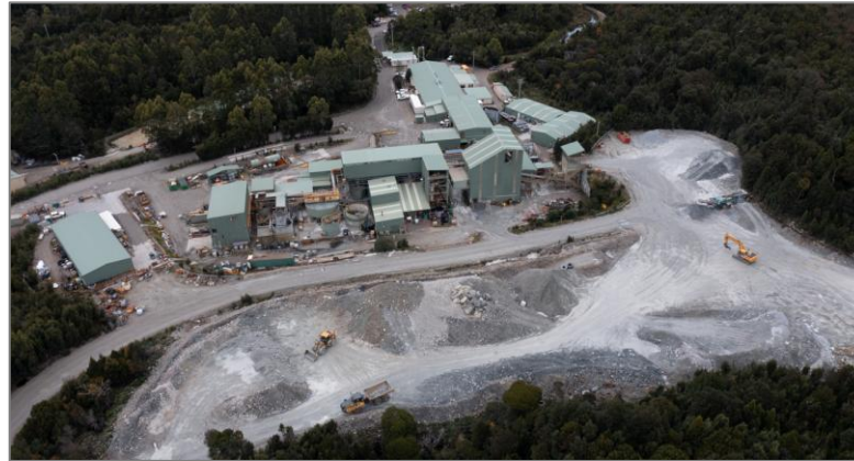
300ktpa CIL Plant & Administration Complex
