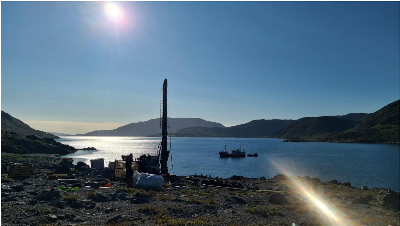
Picture 1 – Drill hole A1-24 September 2024
