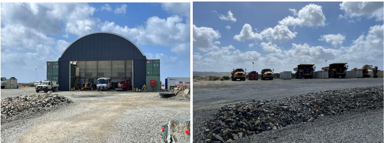
Figure 13 Workshop and Laydown area
