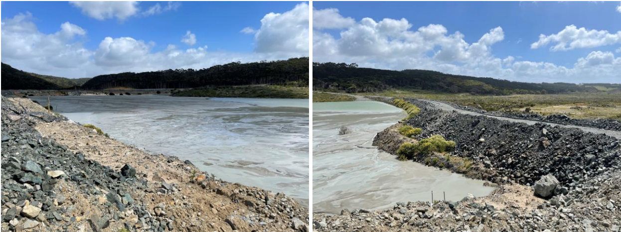
Figure 15 Tailings Storage Facility
