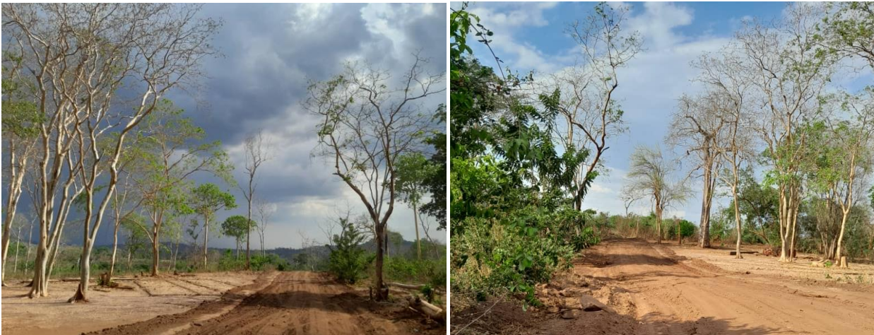
Initial access road clearing at Chilalo
