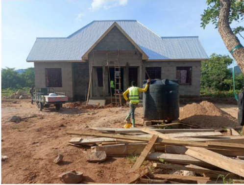
Police station under construction
