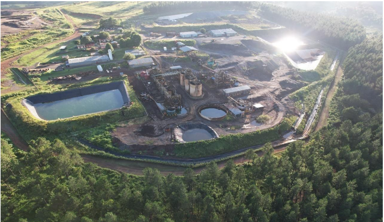
Figure 8: Existing Plant Drone View (post demolition of old sections)
