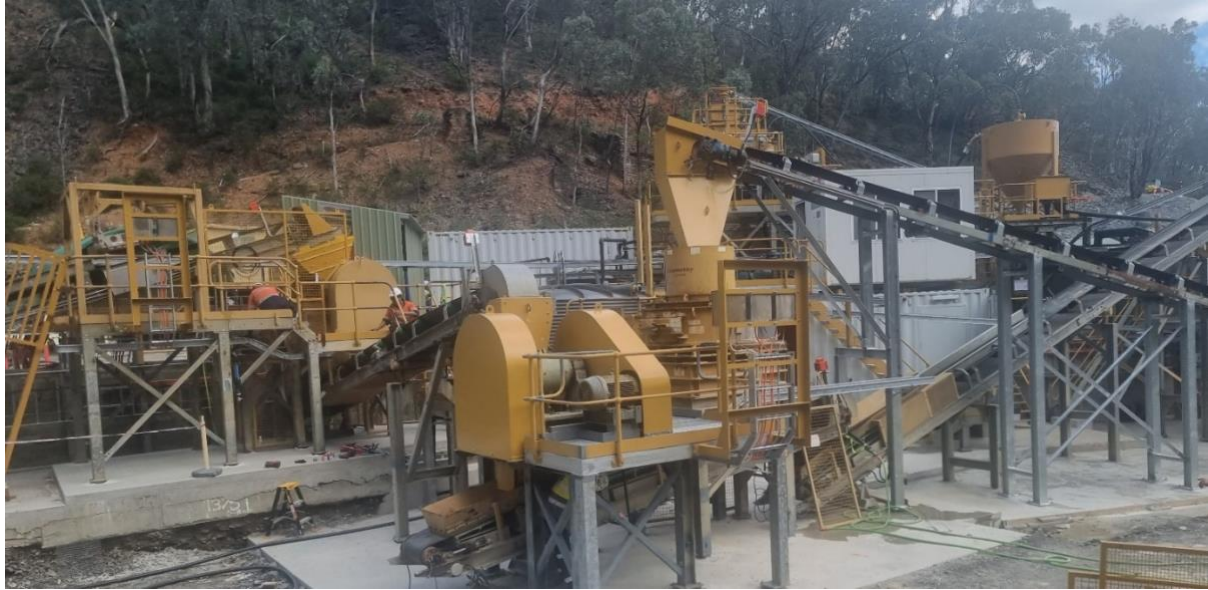
Figure 6 Reward gravity gold plant looking over the 2 jaw crushers and the impact crusher
