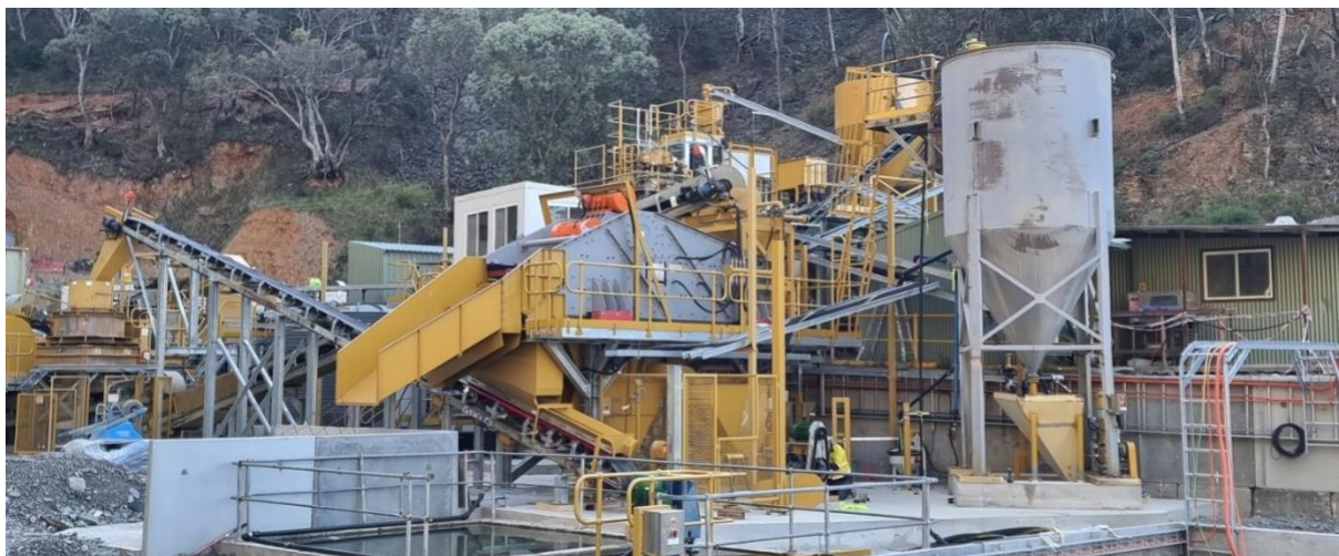
Figure 5 Reward gold gravity plant looking back over the crushing circuit
