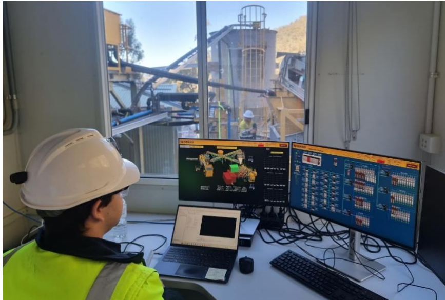
Figure 1 Automation programming technician testing the Reward gravity plant systems from the control room
