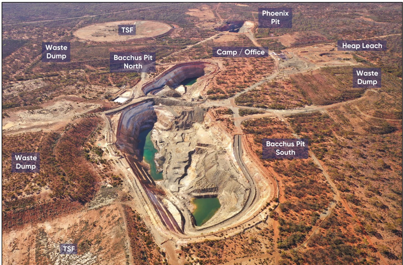
Figure 2 – Image looking north showing former Bullabulling open pits and surface infrastructure
