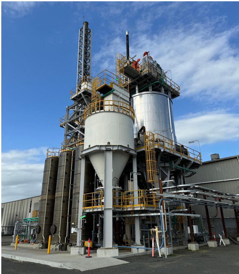
Figure: Spray Roaster reactor vessel insulation works completed
