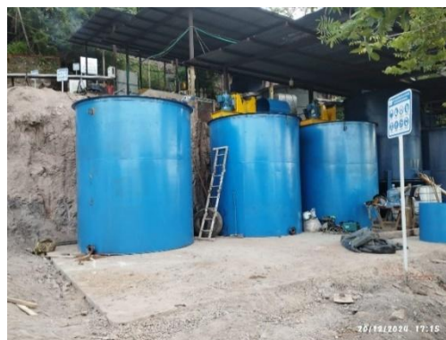
PHOTO 2 : NEW AGITATOR TANKS - SANTA BARBARA PROCESSING PLANT
