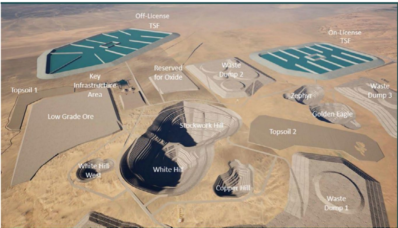
Figure 4-5: Kharmagtai project overview looking north (Xanadu Mines Ltd, 2024e)
