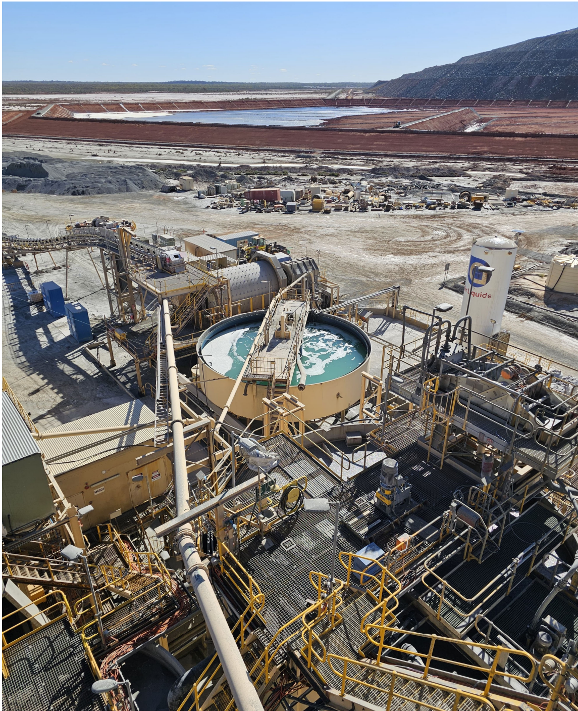
Figure 1: Lakewood processing facility.
