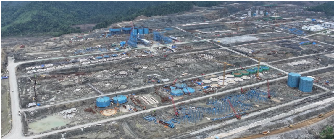
ENC HPAL construction progressing well
