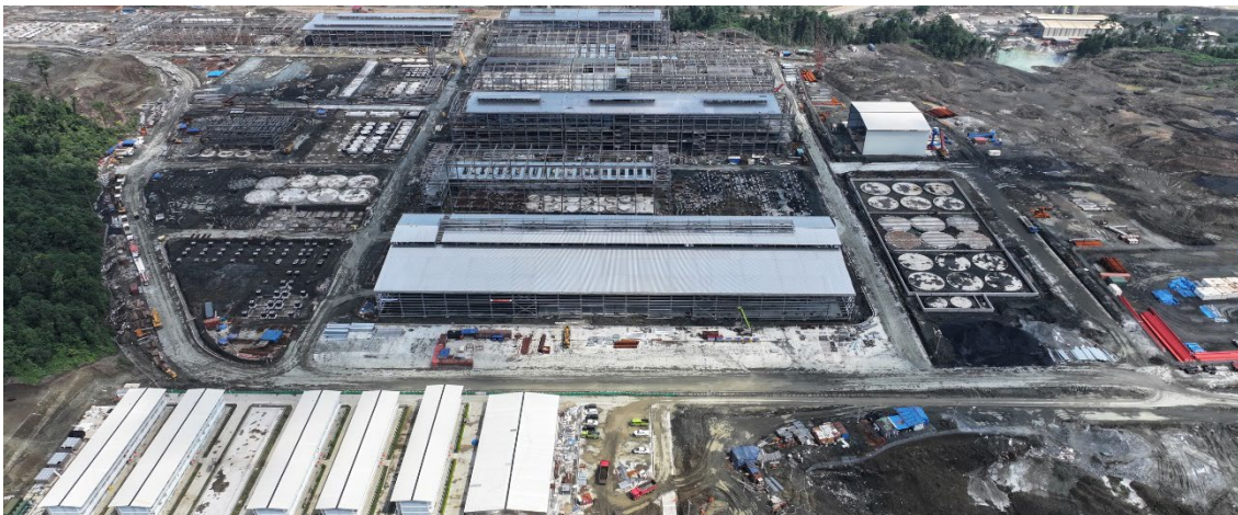
ENC sulphate and cathode refinery construction ahead of schedule
