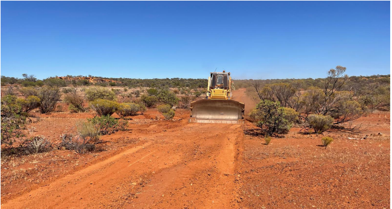
Figure 1: Site works commencing for March drilling program
