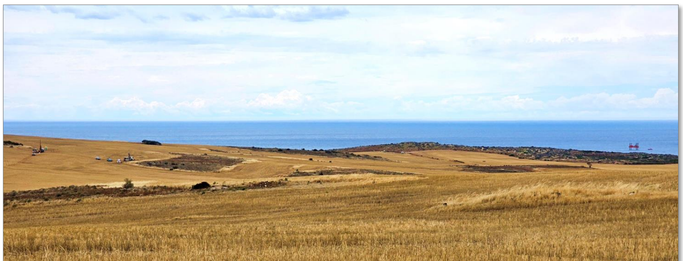
Onshore and offshore geotechnical investigations by Northern Water at the Cape Hardy site, involving trenching and diamond drilling utilising surface drill rigs (LHS) and marine diamond drilling utilising a drill rig mounted on a jack up barge (RHS).
