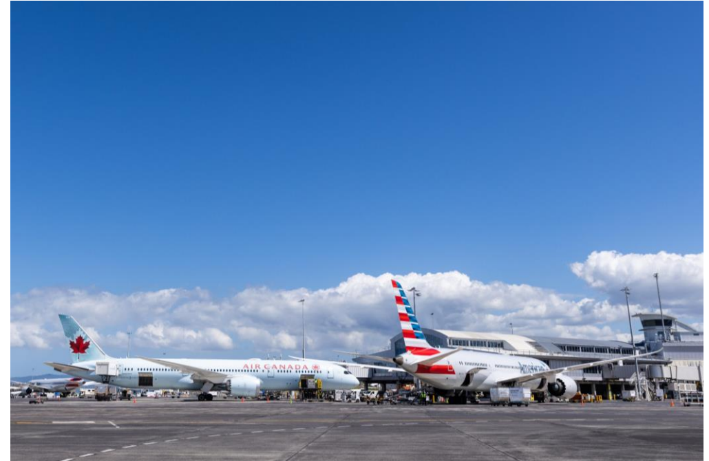
Auckland Airport airfield
