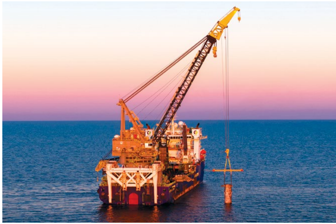
Pictured: Campbell Decommissioning Project
