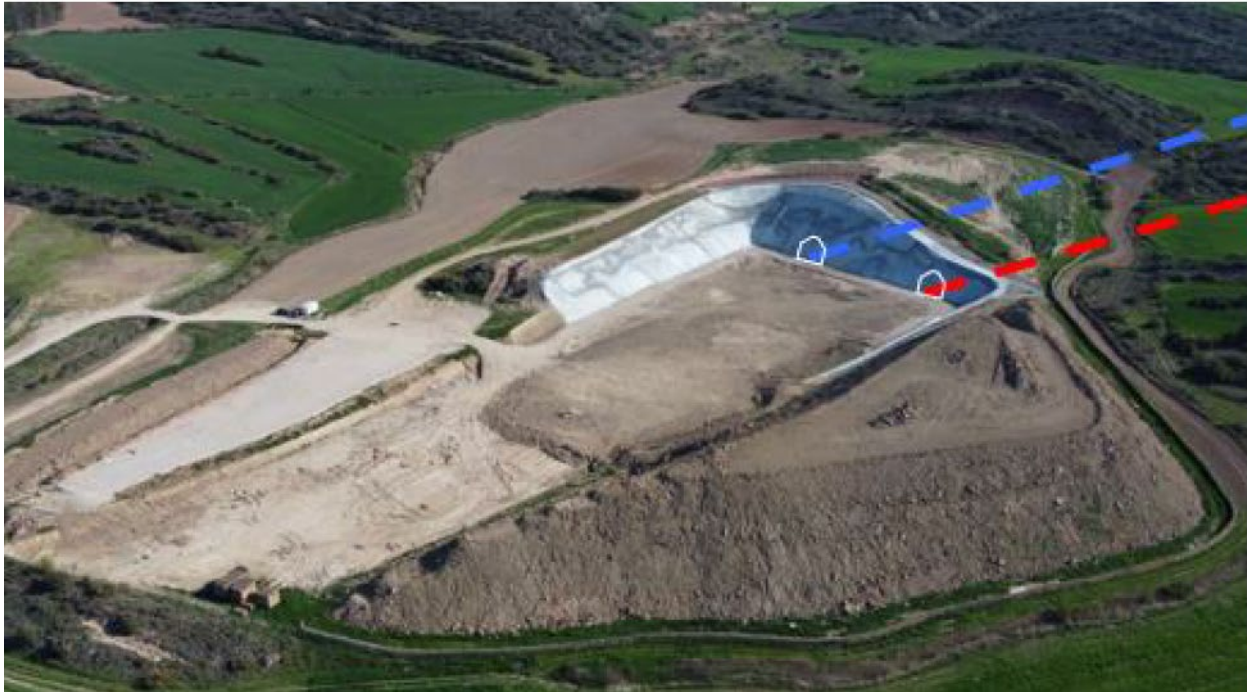
Figure 3-7: Current Status of the Surface Boxcut
