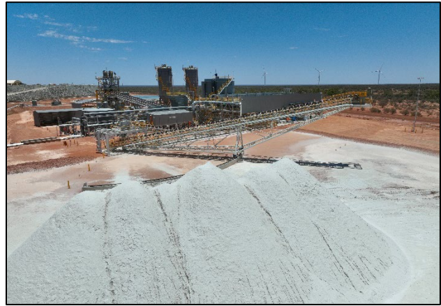
Figure 14: Dry stacking tailings from the paste plant
