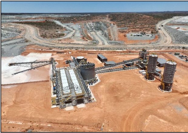
Figure 13: The completed 4Mtpa paste plant
