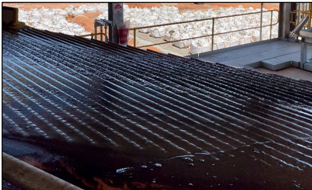
Figure 9: The tantalum circuit in operation
