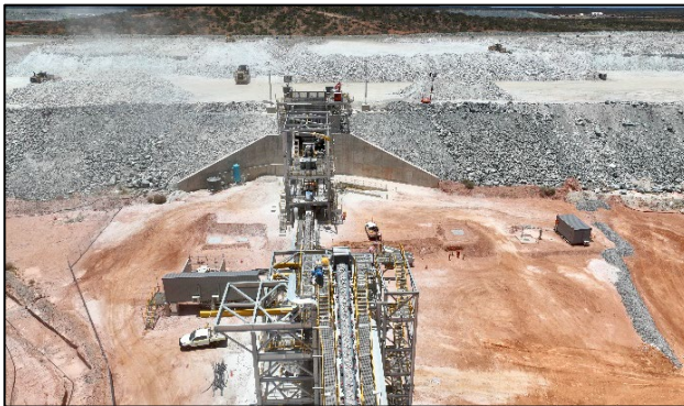
Figure 7: Primary crushing in operation
