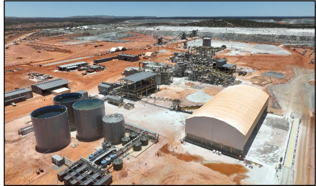
Figure 6: Aerial view of the process plant
