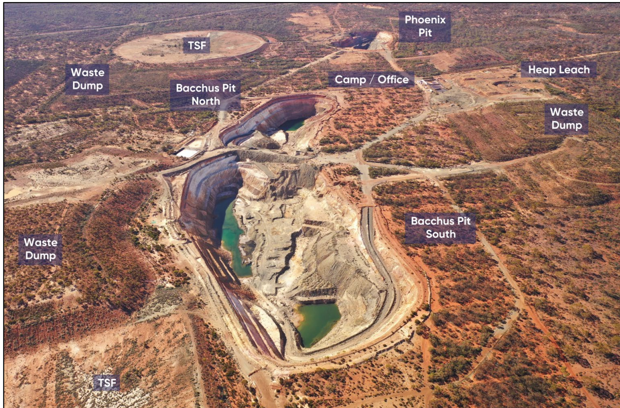
Figure 2 – Image looking north showing historical pits, rehabilitated leach pads and tailings storage facility and exploration camp
