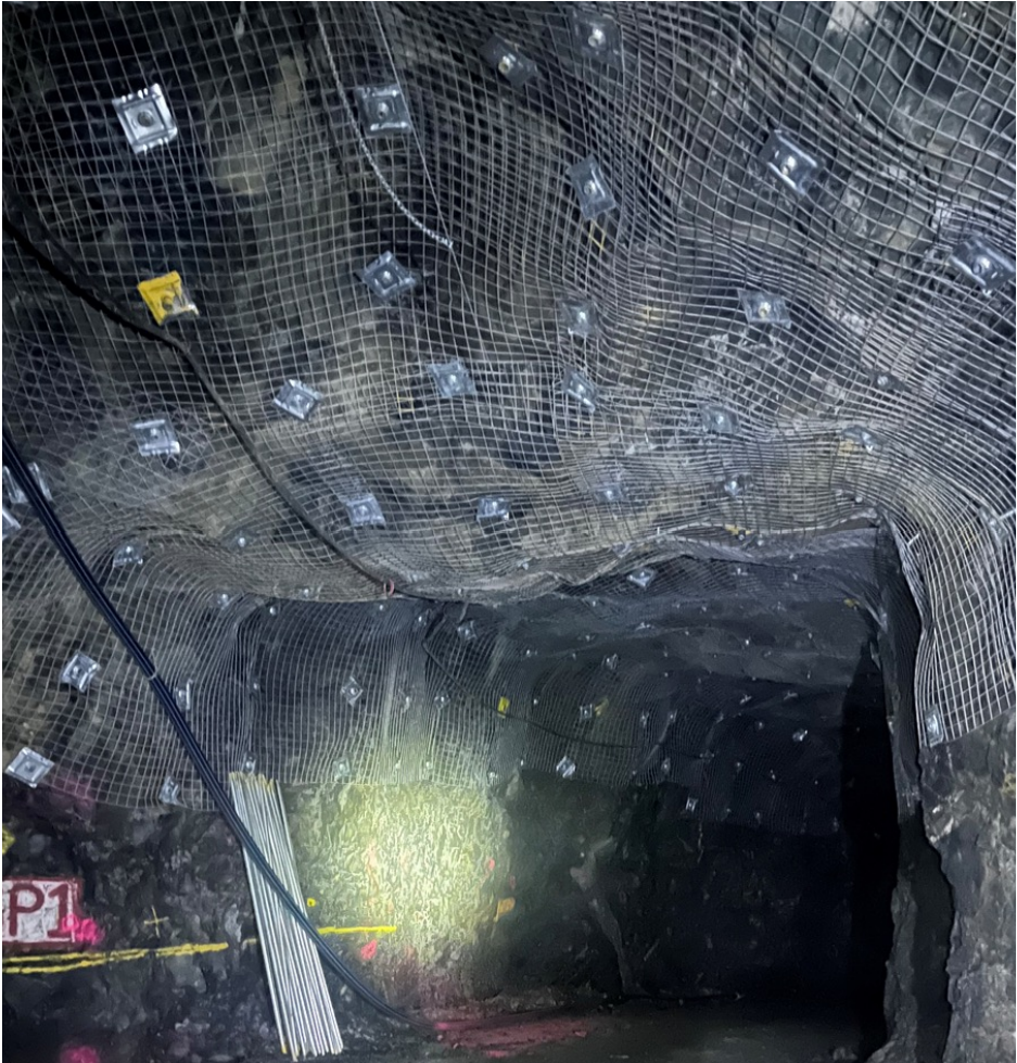
Figure: Ongoing support works showing excellent ground conditions.
