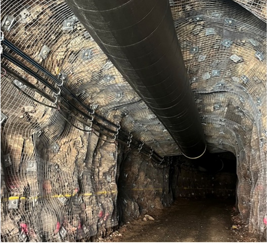
Picture: Full mesh ground support close to the Bullen Portal.
