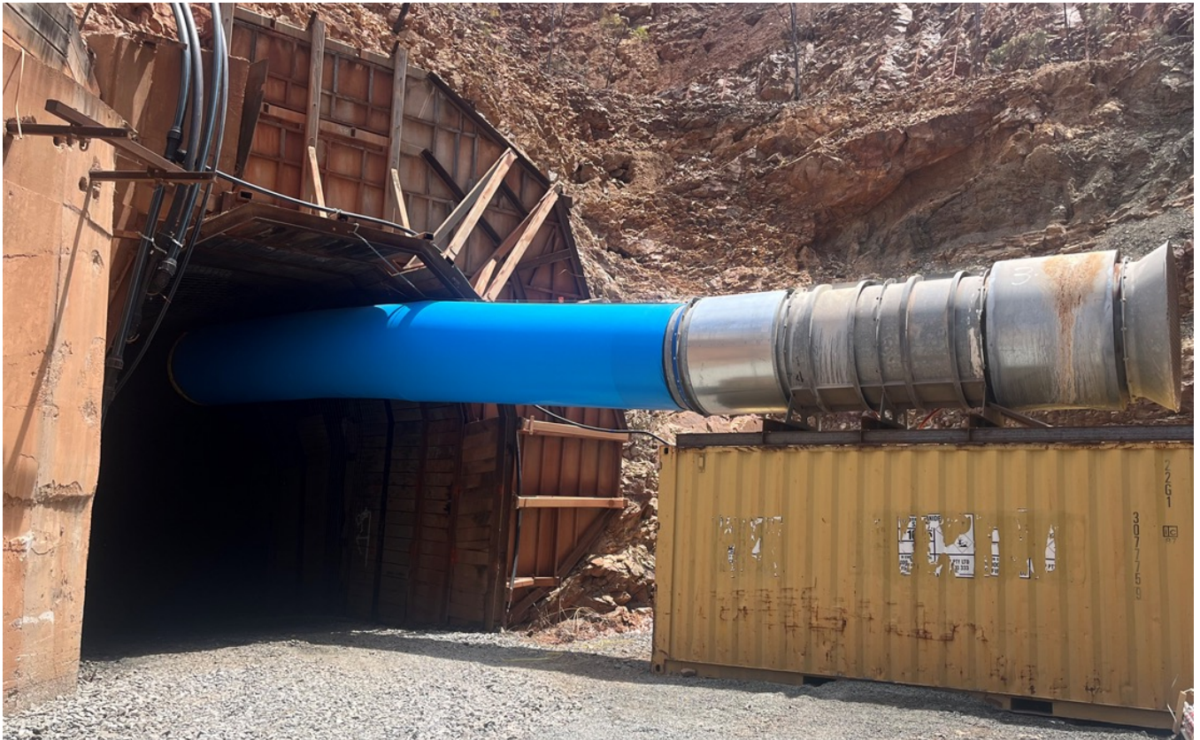
Picture: Temporary ventilation established at the Bullen Portal.
