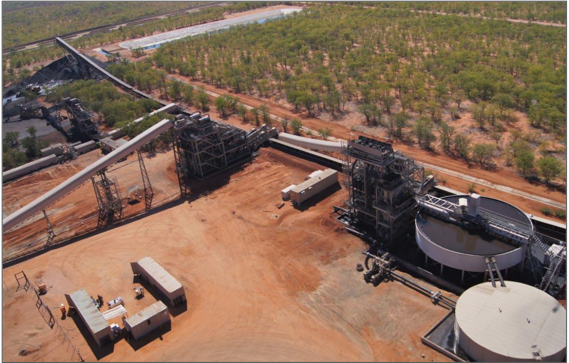
Figure 4.7: Vele wash plant
