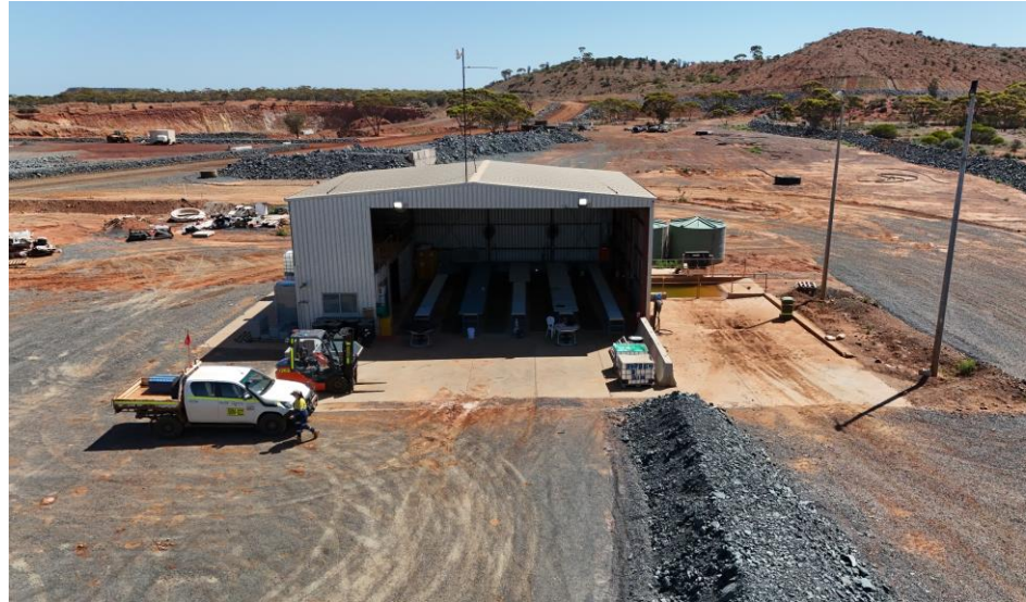
Figure 15 - Sand King – on site core processing facility
