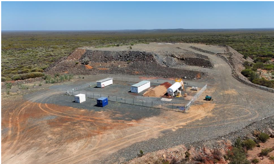
Figure 16 - Explosive and emulsion magazine
