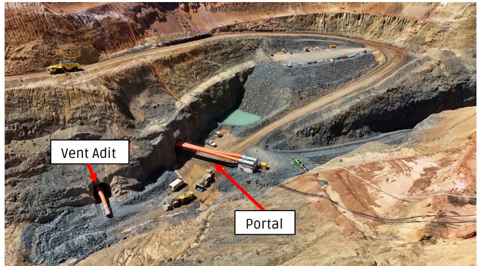
Figure 13 - Sand King Portal and newly established ventilation adit
