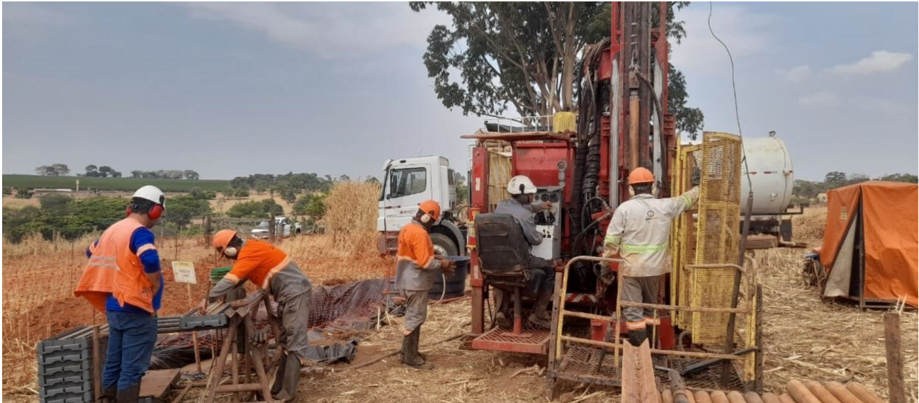
Figure 6: Diamond Drilling Progressing at Mata da Corda
