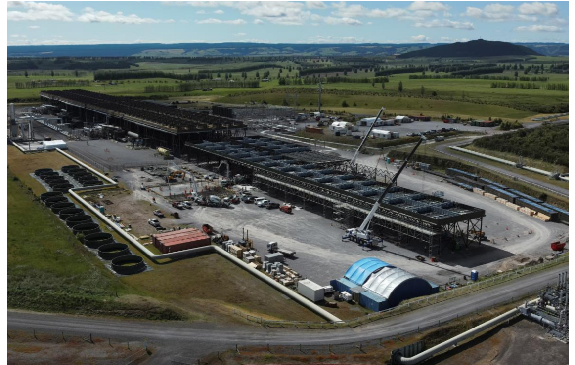
Ngā Tamariki OEC5 geothermal under construction
