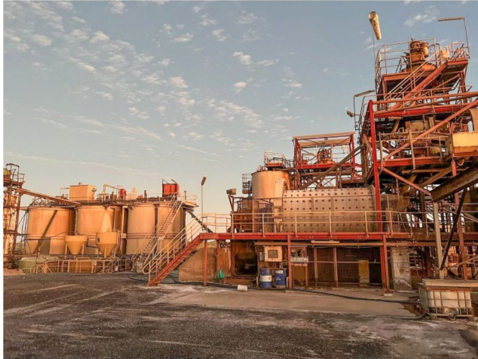
Figure 2 – Lorena Processing Facility
