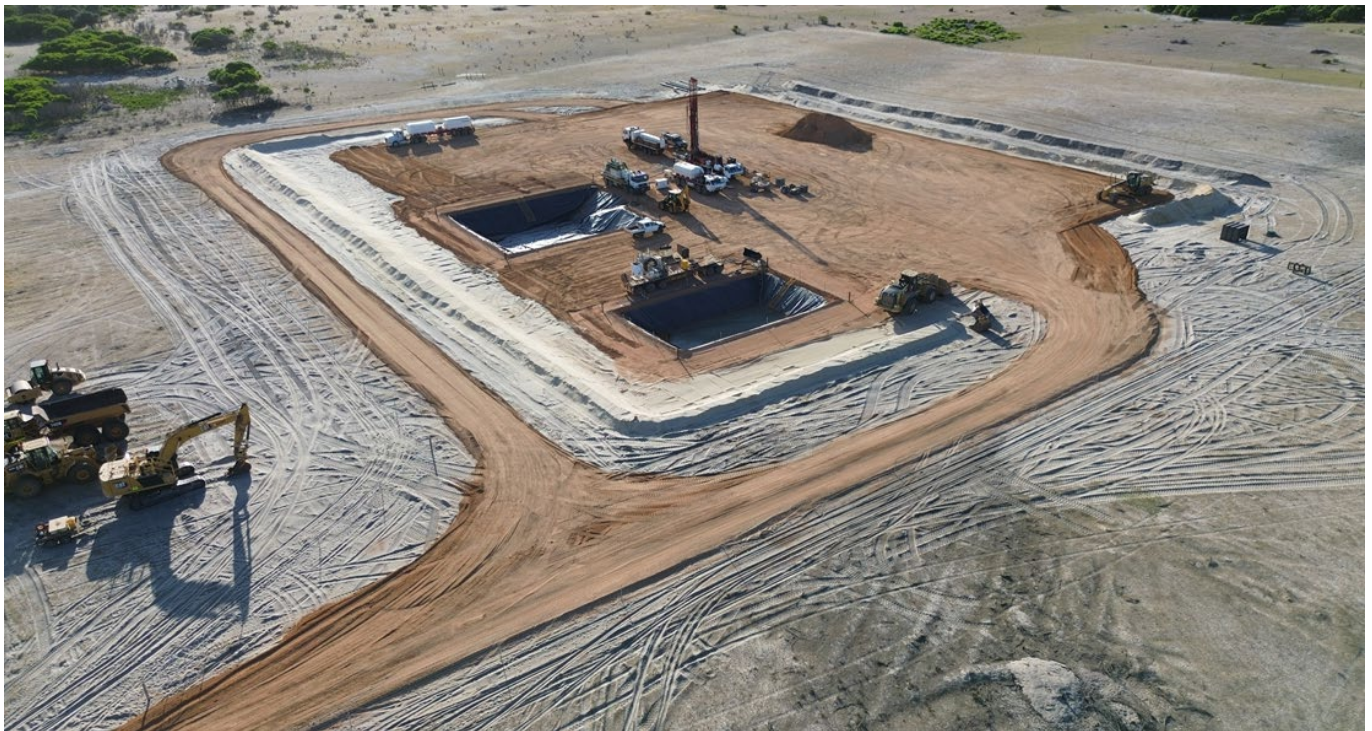
Figure 1: Becos-1 well pad nears completion
