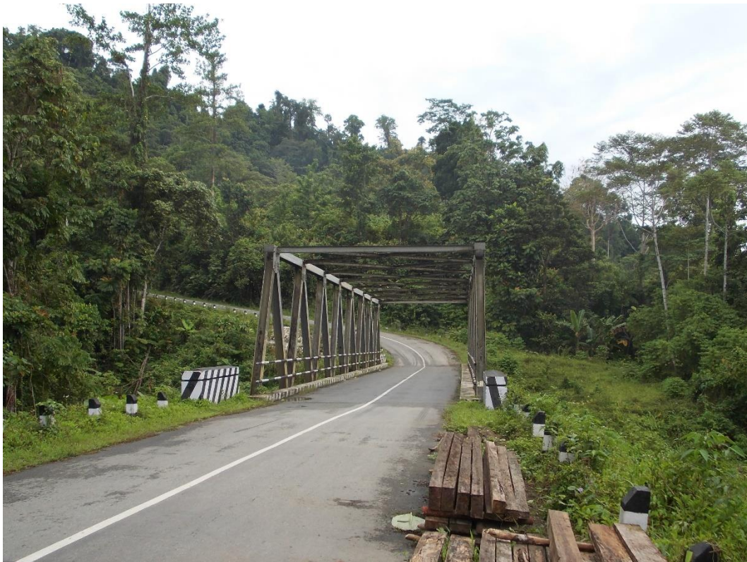
Figure 1.6 – Bridge 120 kilometres from the Concession
