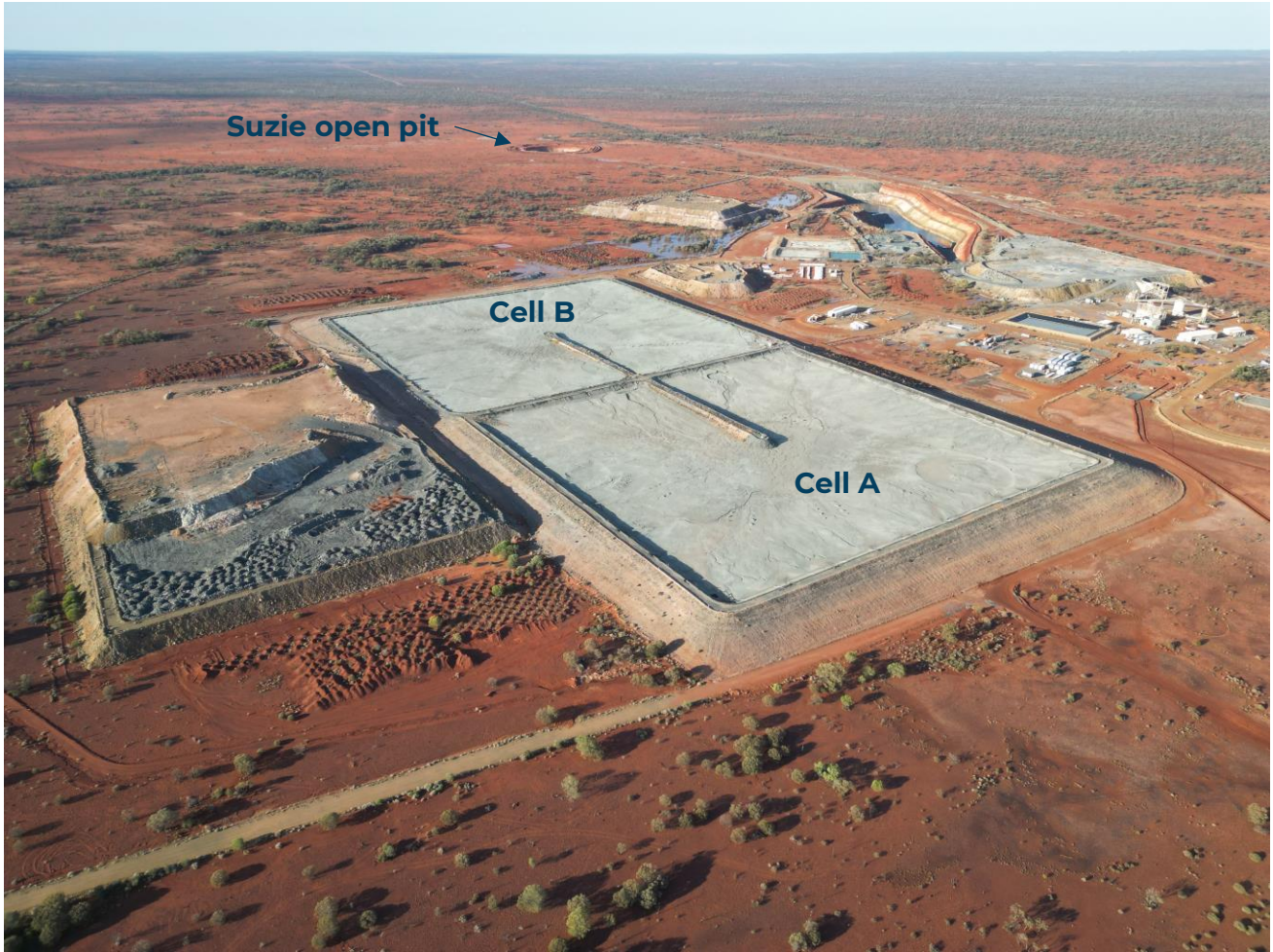
Figure 42 – Existing TSF, December 2024.
