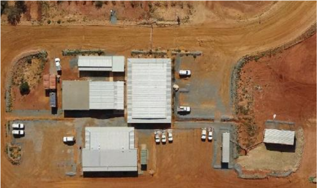
Figure 48 – Andy Well Administration (to be reinstated during site establishment phase).
