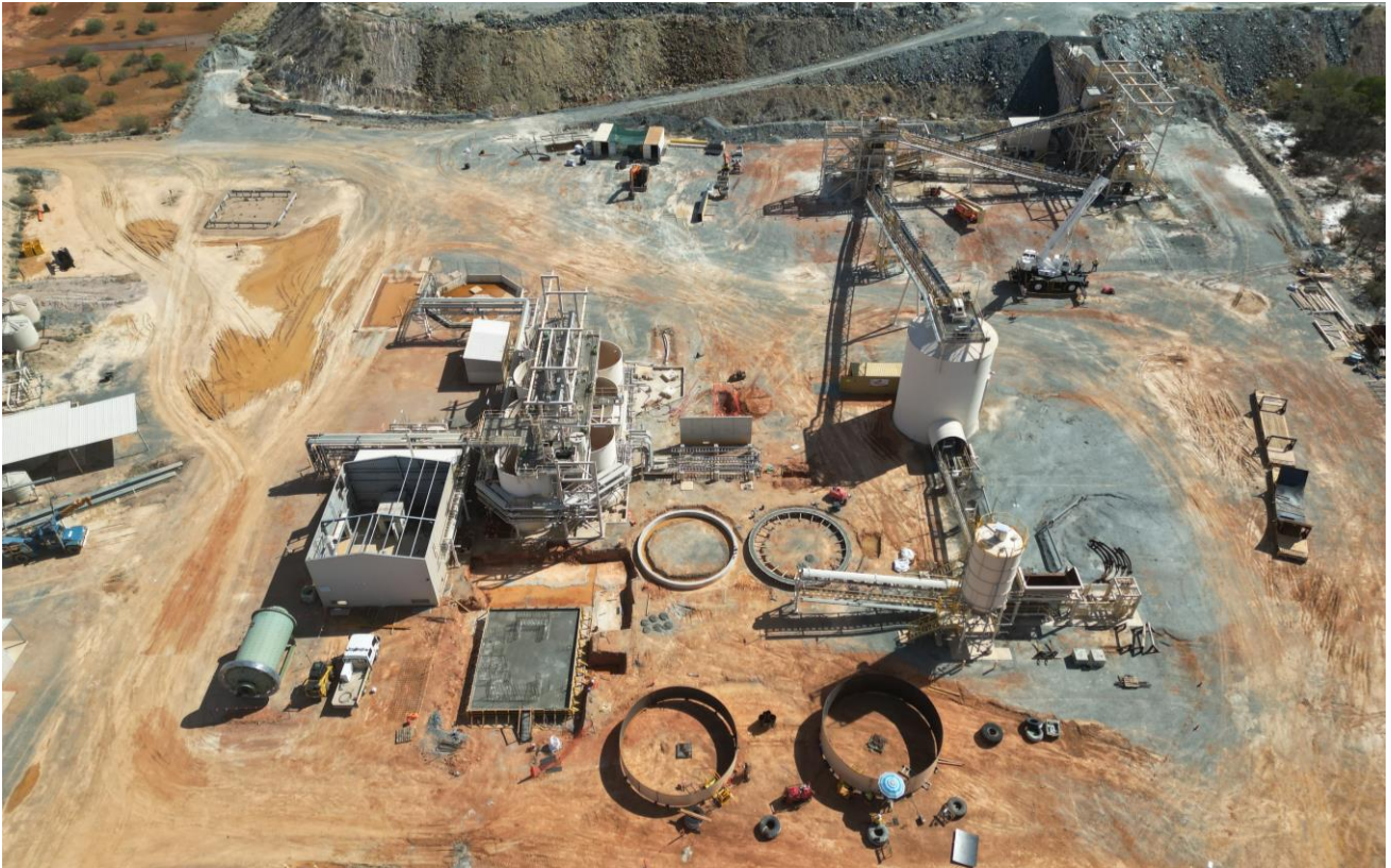
Figure 41 – View of the new leach and adsorption tank foundations and tank skins being fabricated (November 2024).
