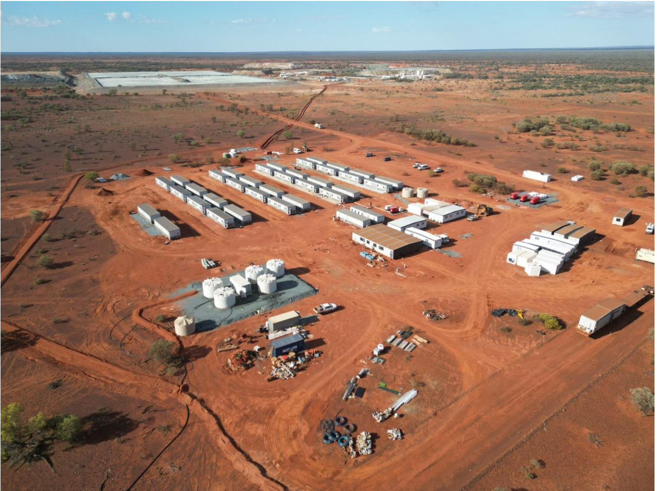
Figure 49 – Andy Well 136-person accommodation village and associated infrastructure.
