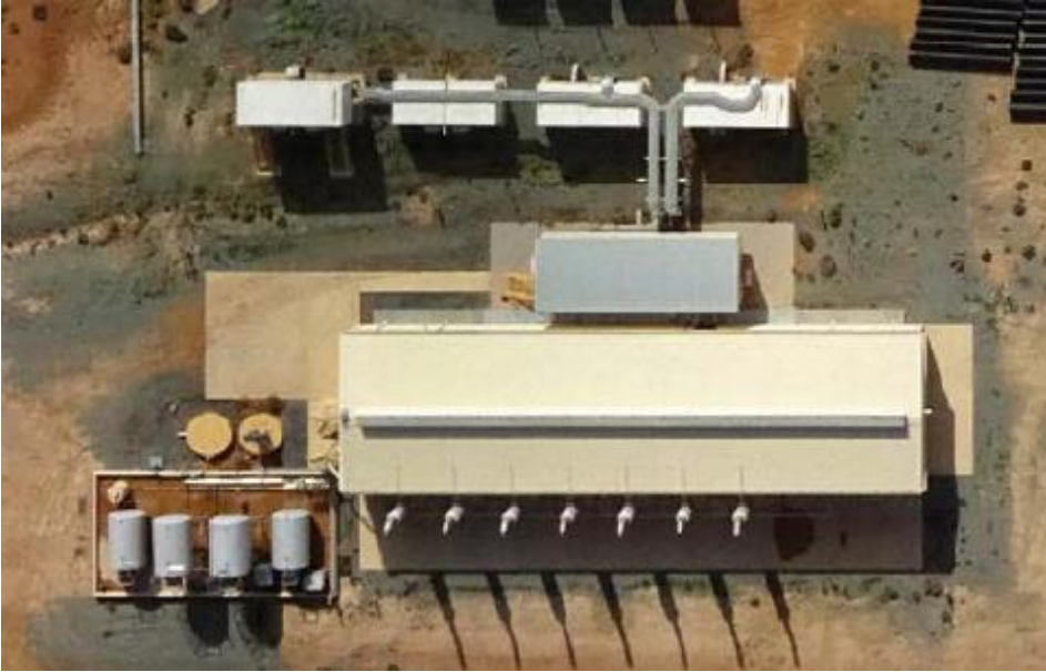
Figure 52 – Andy Well power station.
